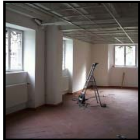
The new Ceiling
